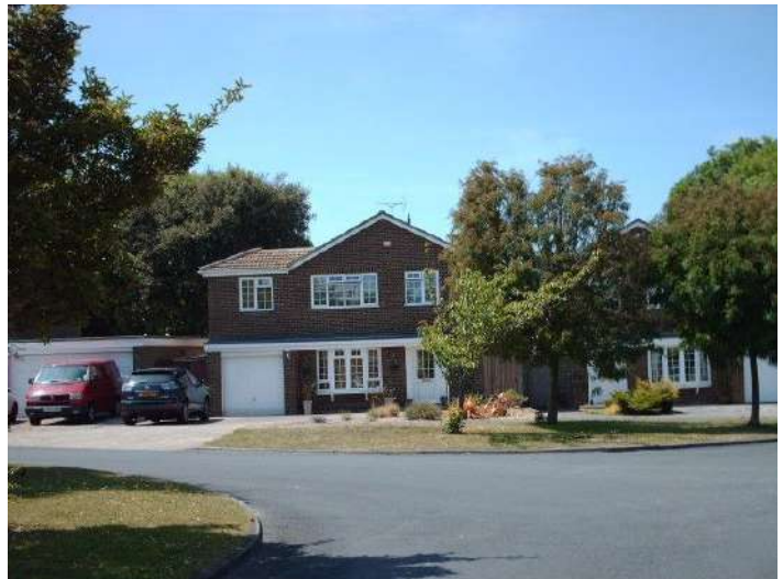
Sympathetic garage extension
