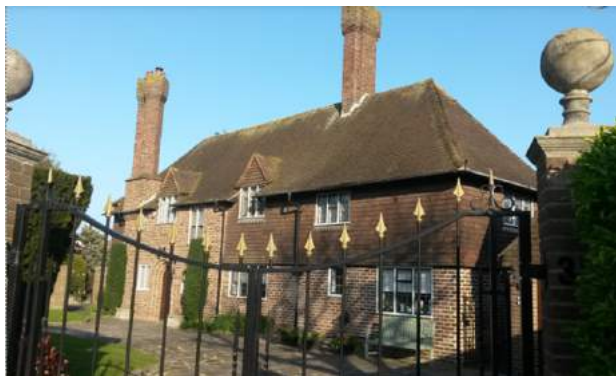
3 Waldron Road (Crossways)
