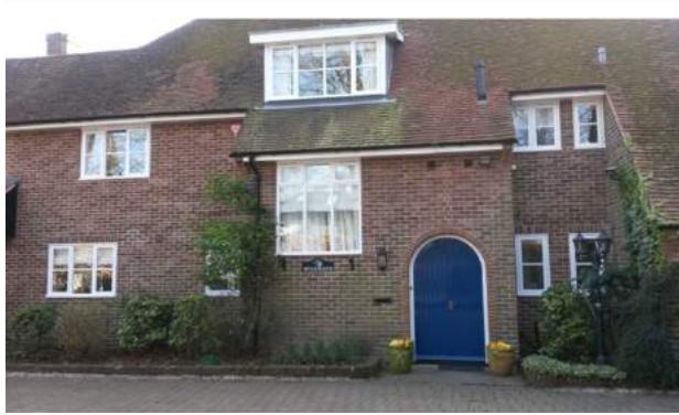
4 Fig Tree Road (Woodgate)
