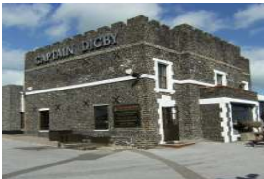
Captain Digby Public House Grade II Listed
