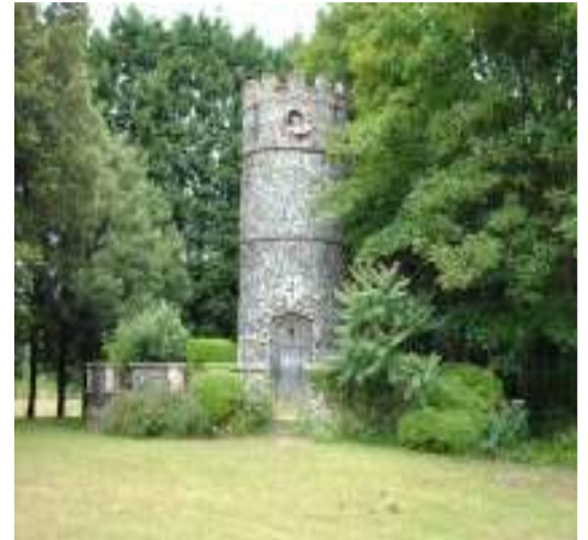
Hackemdown Tower (within Port Regis) Grade II Listed
