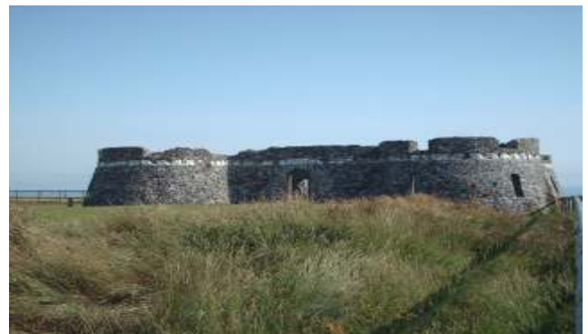
Remains of Neptune's Temple, Kingsgate Grade II Listed
