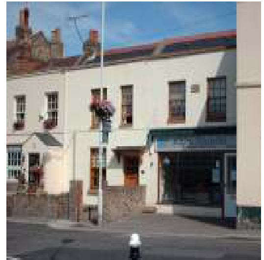
Sympathetic New Build Church Street St. Peter's
