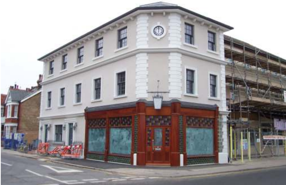
An excellent example of new build – Broadstairs High Street, completed 2011
