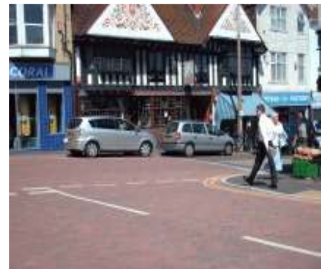
High Street - New Block Paving
