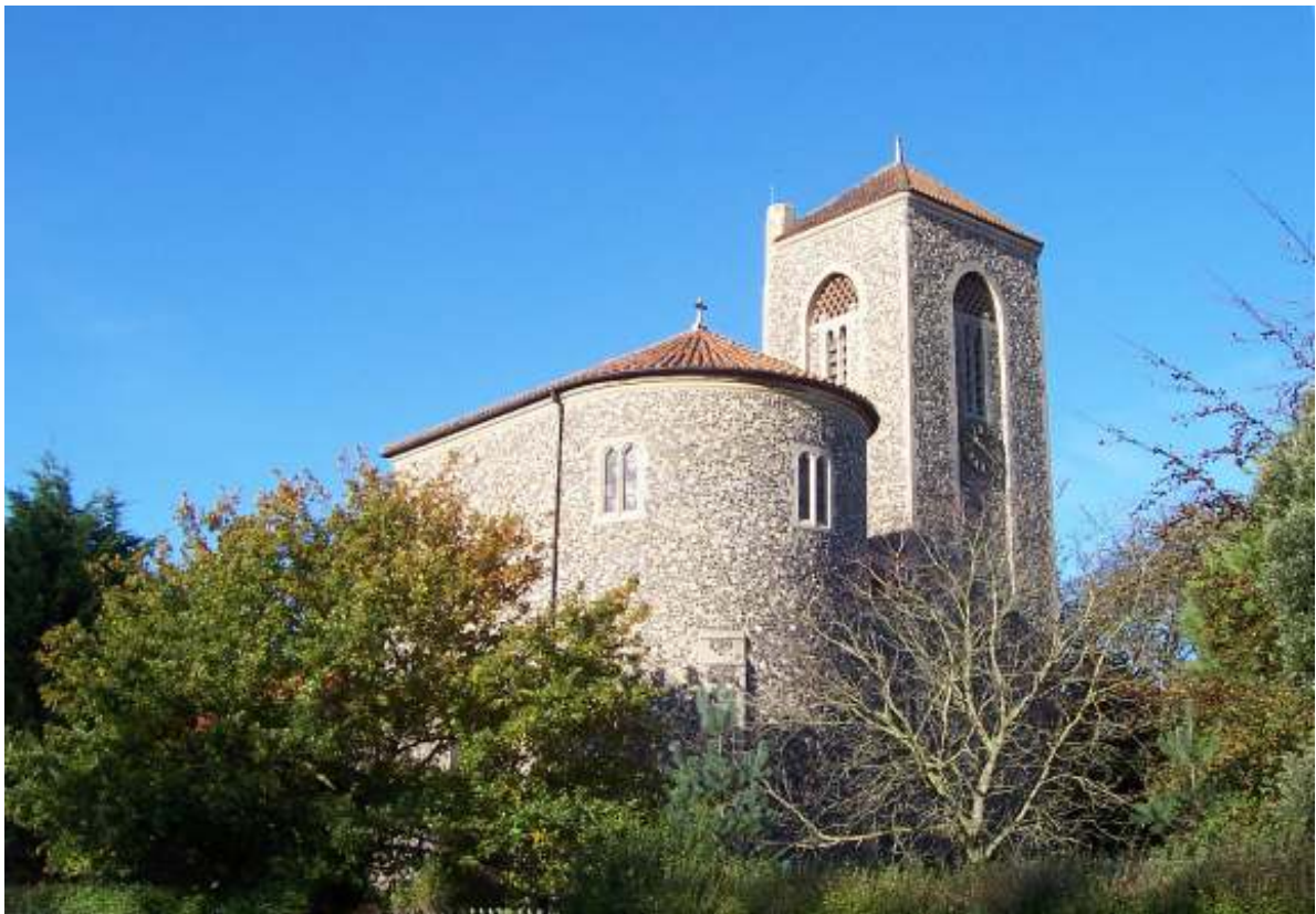
Roman Catholic Church of Our Lady Star of the Sea, Broadstairs Road Grade II Listed. 1930-1, by Sir Giles Scott, completed 1961. Flint with stone dressings, pantiled roof.
